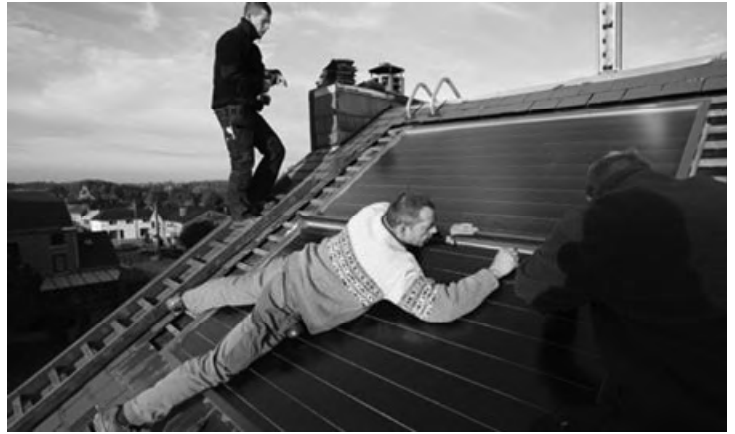
Installing solar panels
